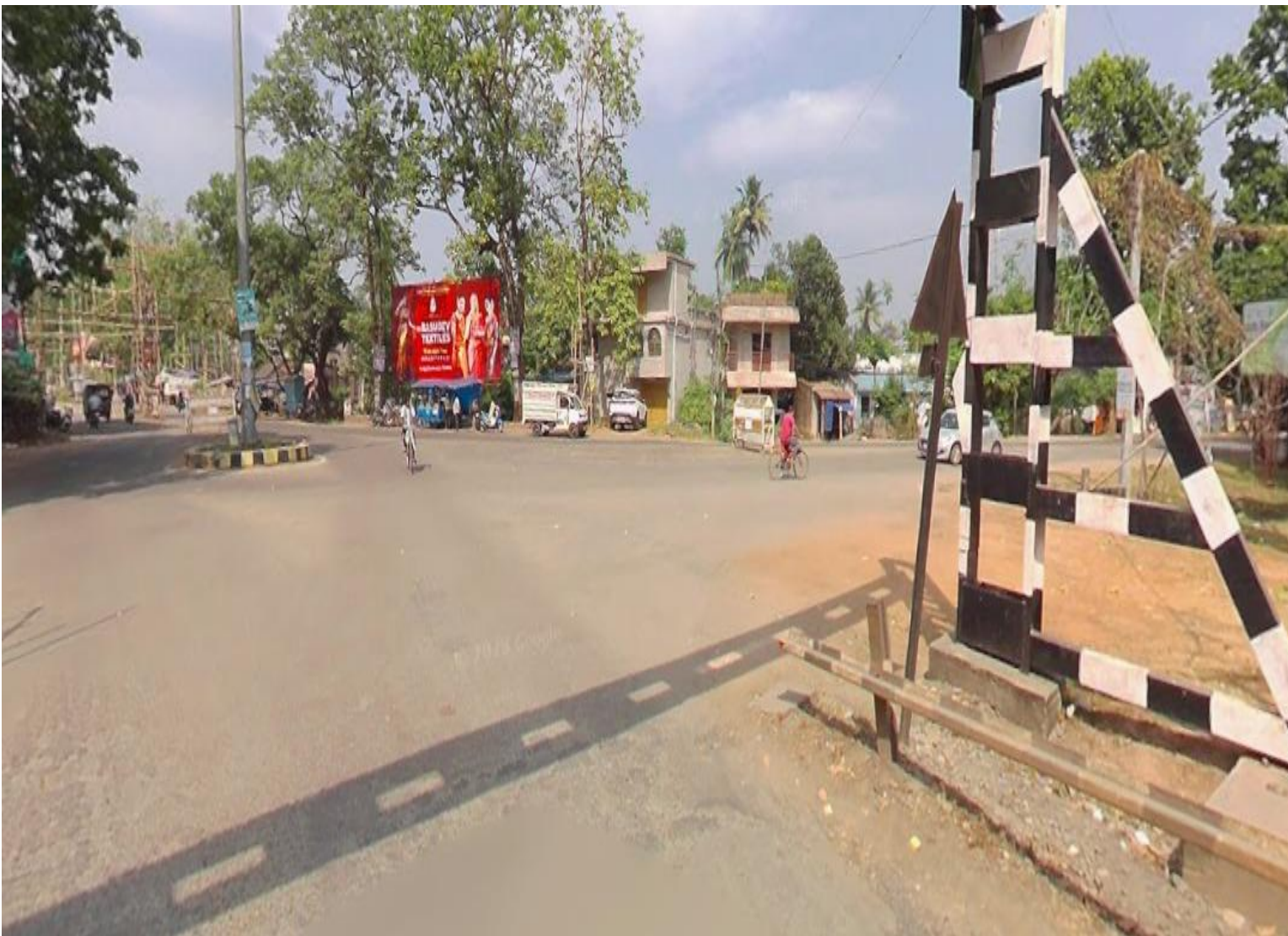
IMAGE: RAILWAY CROSSING ;RiskLevel: MEDIUM ;Coordinates: 21.9199201,86.7435814 (60.3 km)
